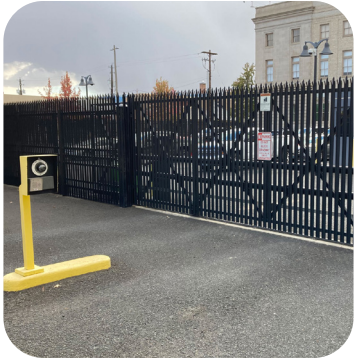
GATES / ACCESS CONTROL
